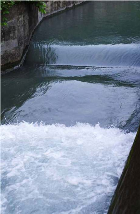
Figure 1. Hydraulic jump in a man-made water supply channel in November 2010.
