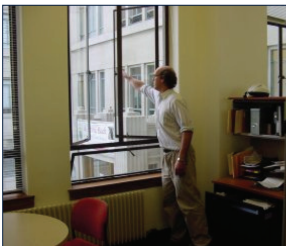
Figure 2a. An office in the naturally ventilated building (Berkeley Civic Center, California)
