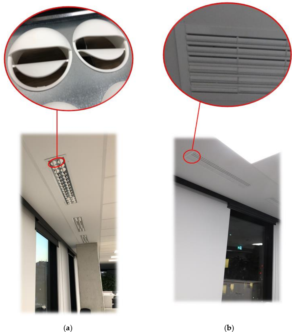
Figure 2. Linear diffuser: (a) Type I; (b) Type II.
