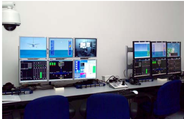
Figure 8. Operations Engineering Station (left) and Operations Command Station in BRS
