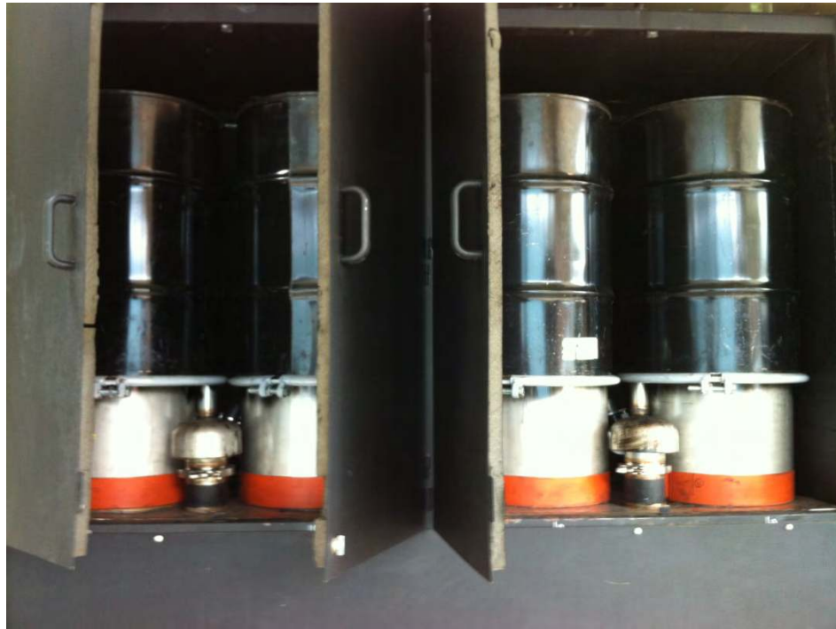
Figure 9-12: Filter box with doors open. Bags are inverted inside barrels by syngas flow
