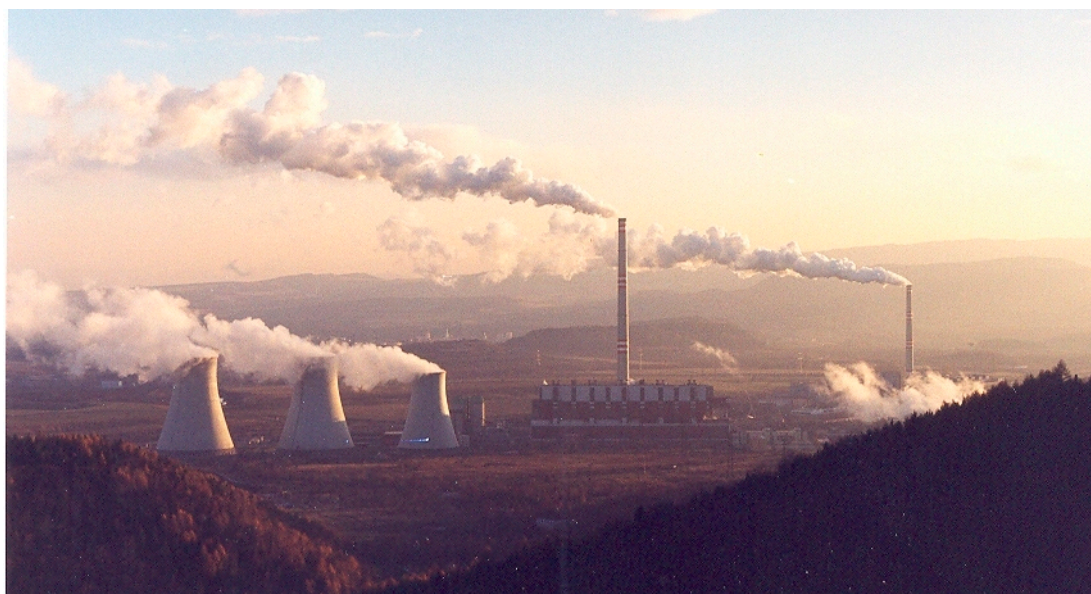
Figure 1. Prunerov coal power plant (photo by the author).
