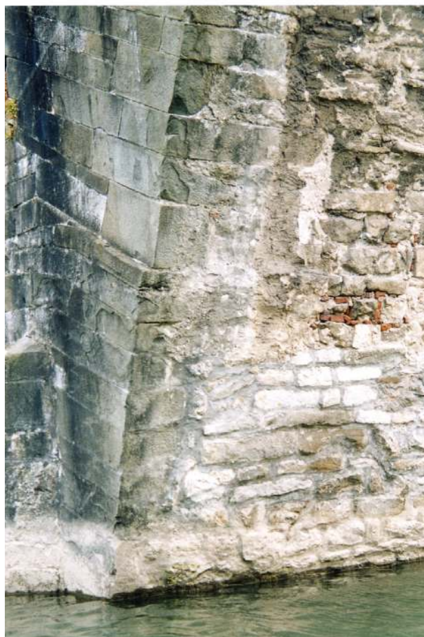
Figure 3. Detail of the masonry texture on the main arch: at the left haunch on the downstream side (top) and at the left springer on the upstream side (bottom).
