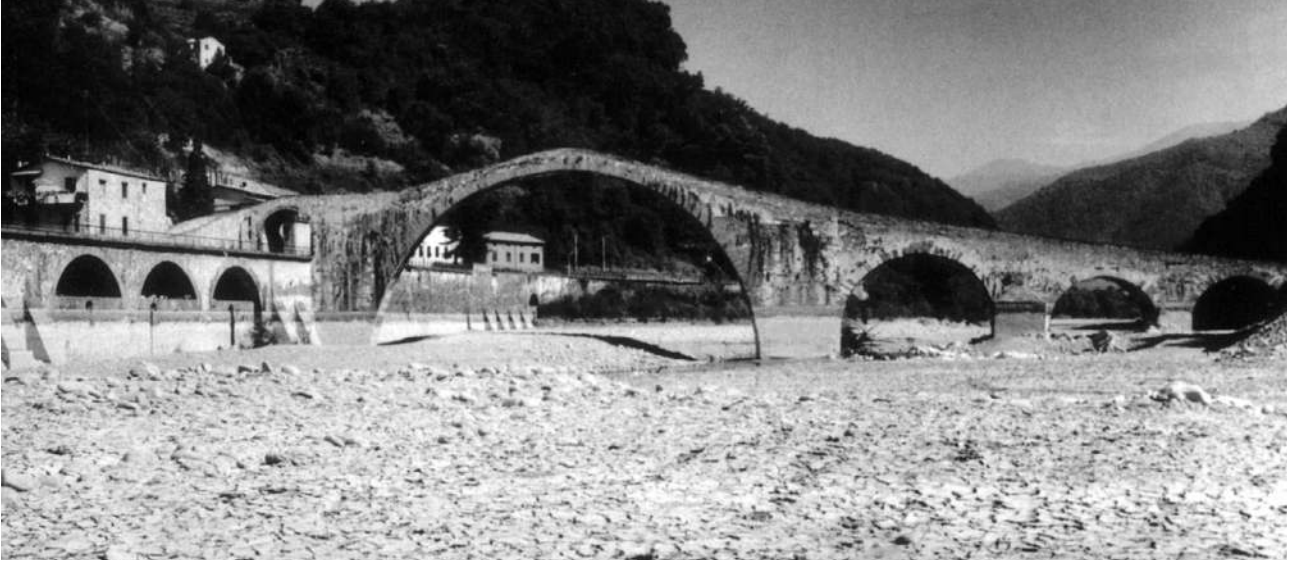
Figure 1. The Maddalena Bridge and adjacent railway.
