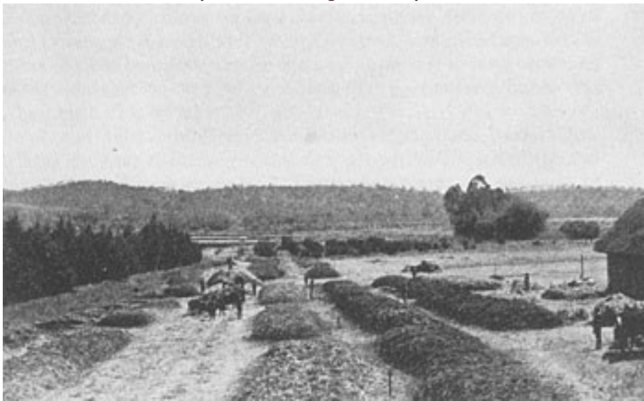
General view of composting area.
