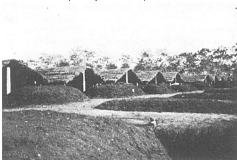
Covered and uncovered pits.
