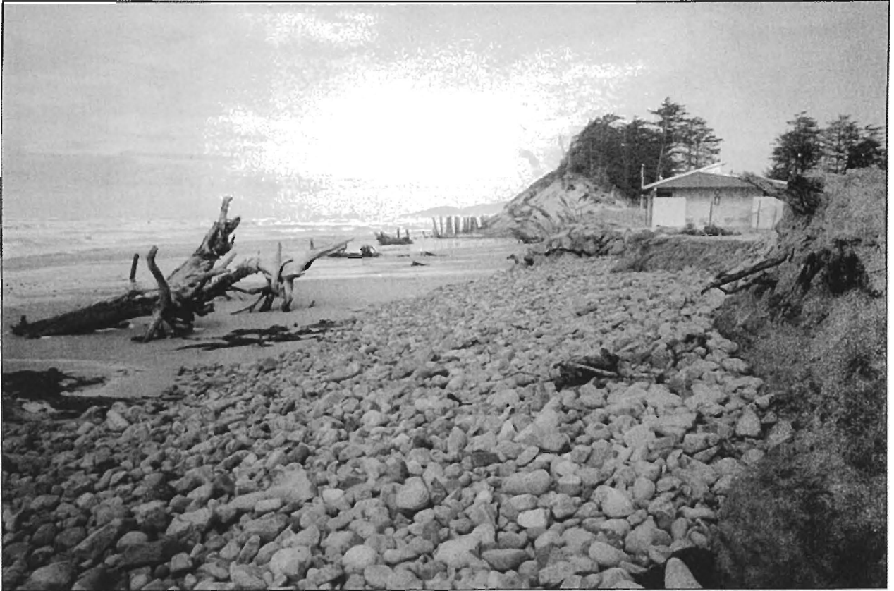
Figure 3. Erosion in Cape Lookout State Park during the 1997–98 El Niño. Remnants of the log seawall can be seen in the background, together with the eroding high dunes. The bathrooms were threatened, and had to be protected by a line of riprap (Photo: Komar).
