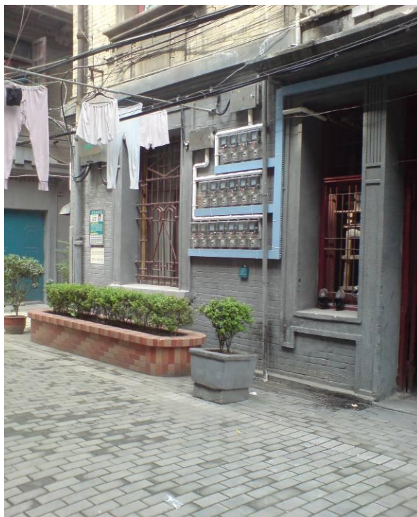
Figure 54 Meter boxes after upgrading, 2008
