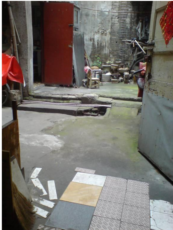
Figure 59 Upgrading against flooding in the backyard
