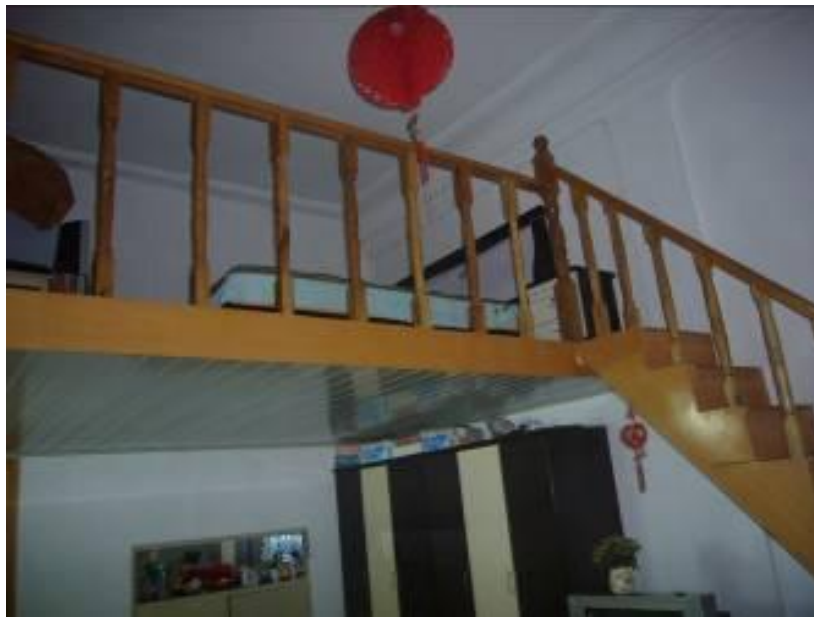
Figure 47 Typical inserted mezzanine
