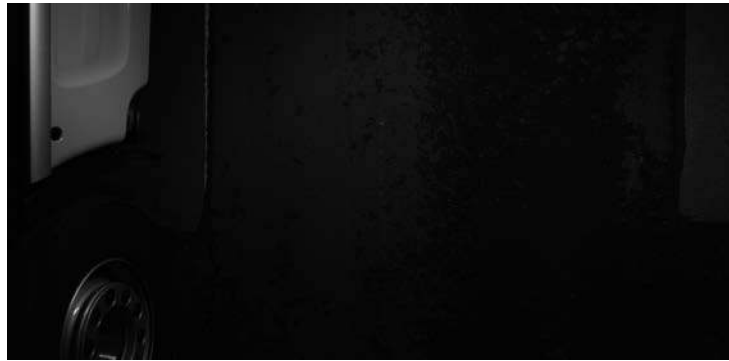
Figure 6.14: Image with low pavement texture, shadows from vehicles, and oil spots without cracks (LEHMANN+PARTNER 2014).
