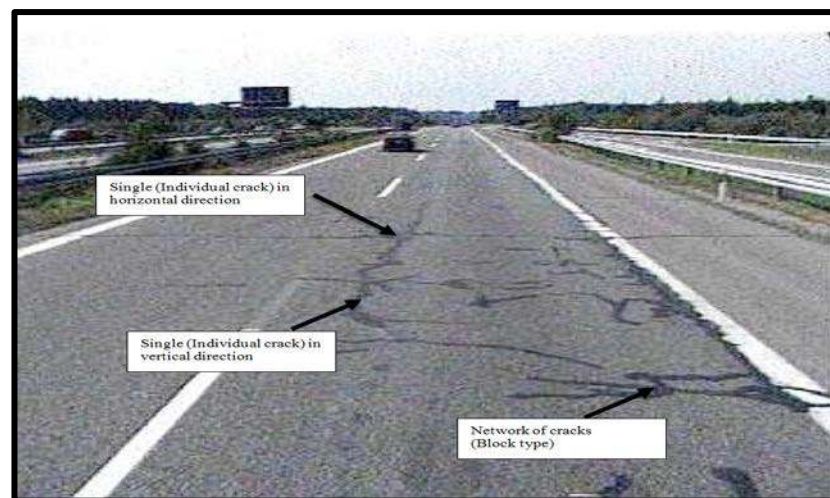
Figure 2.1: Cracking (FGSV 2006).
