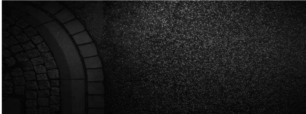
Figure 6.16: Image with high pavement texture and a sidewalk (curb) without cracks (LEHMANN+PARTNER 2014).
