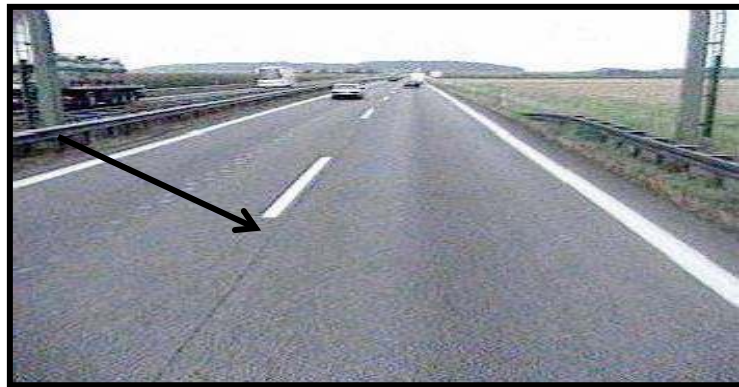
Figure 2.4: Open work seams (FGSV 2006).
