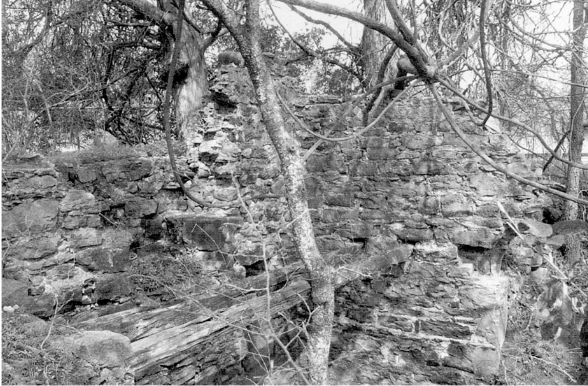
Figure 87. Aussilloux House showing remains of floor joists.
