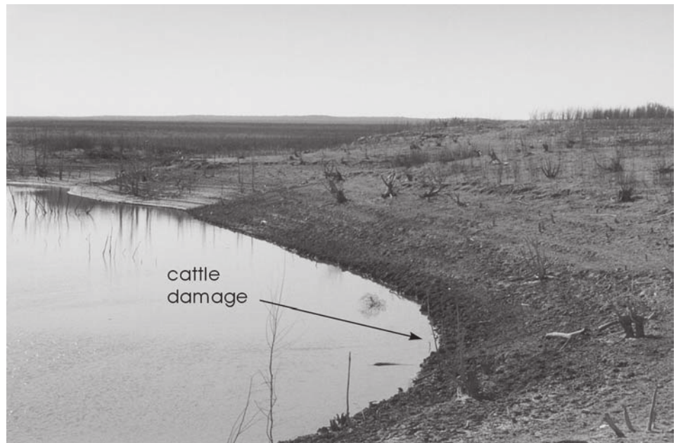
Figure 2-20. Cattle damage along Spring Creek shoreline.
