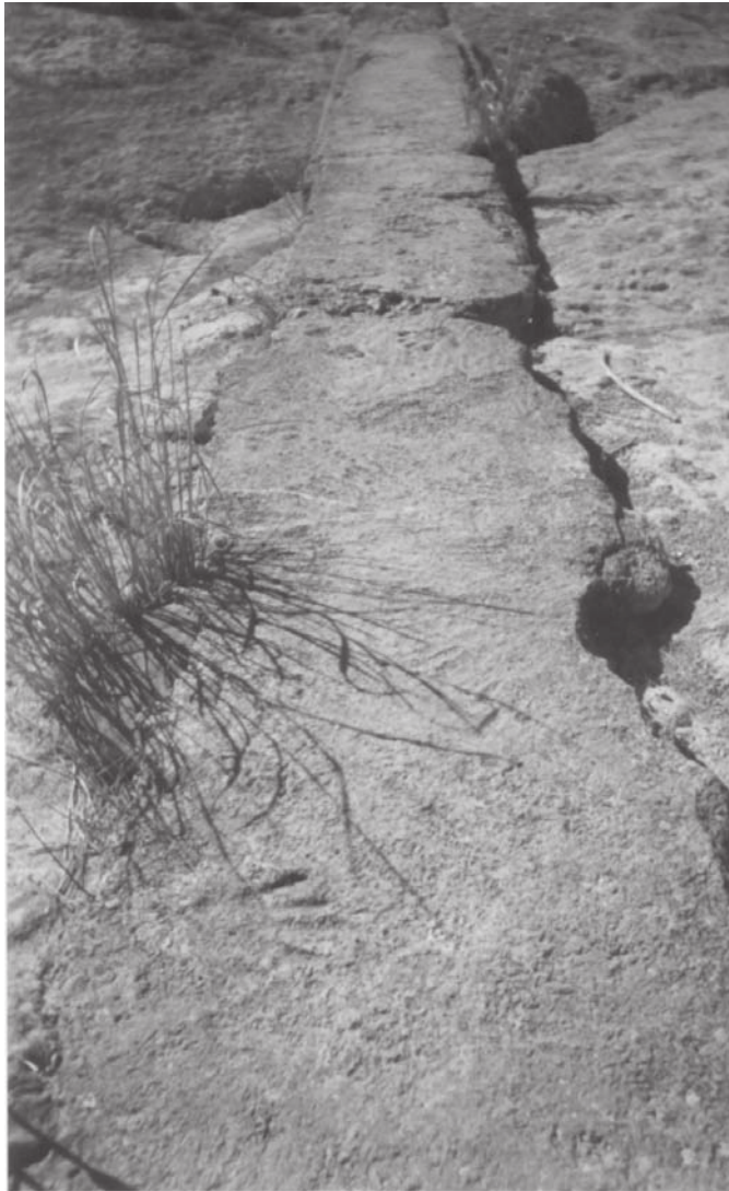
Figure 11-5. Writing and impressions on concrete ditch wall just below White's Dam.
