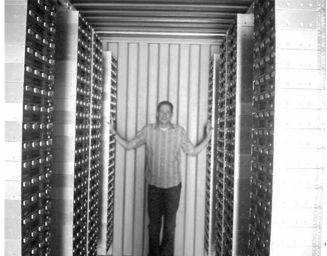
Figure 3: Rackable Systems Data Center in a Box
