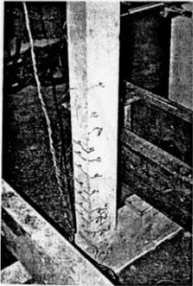
Figure E7. PF2: location E.
