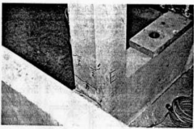
Figure E6. PF1: location E.
