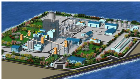
Fig. 1.2 Estimated bird's-eye view of Kwangyang SNG plant [60].
