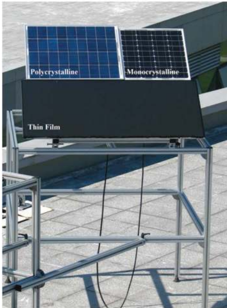
FIGURE 4: The platform with three different PV panel technologies positioned with 41° tilt angle.
