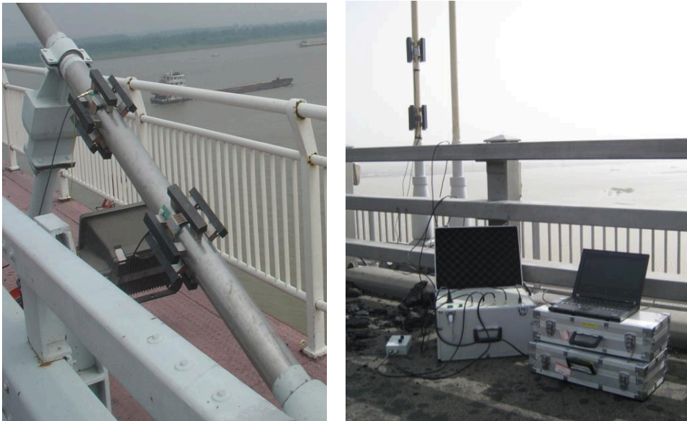
(a) Cable-stayed bridge
