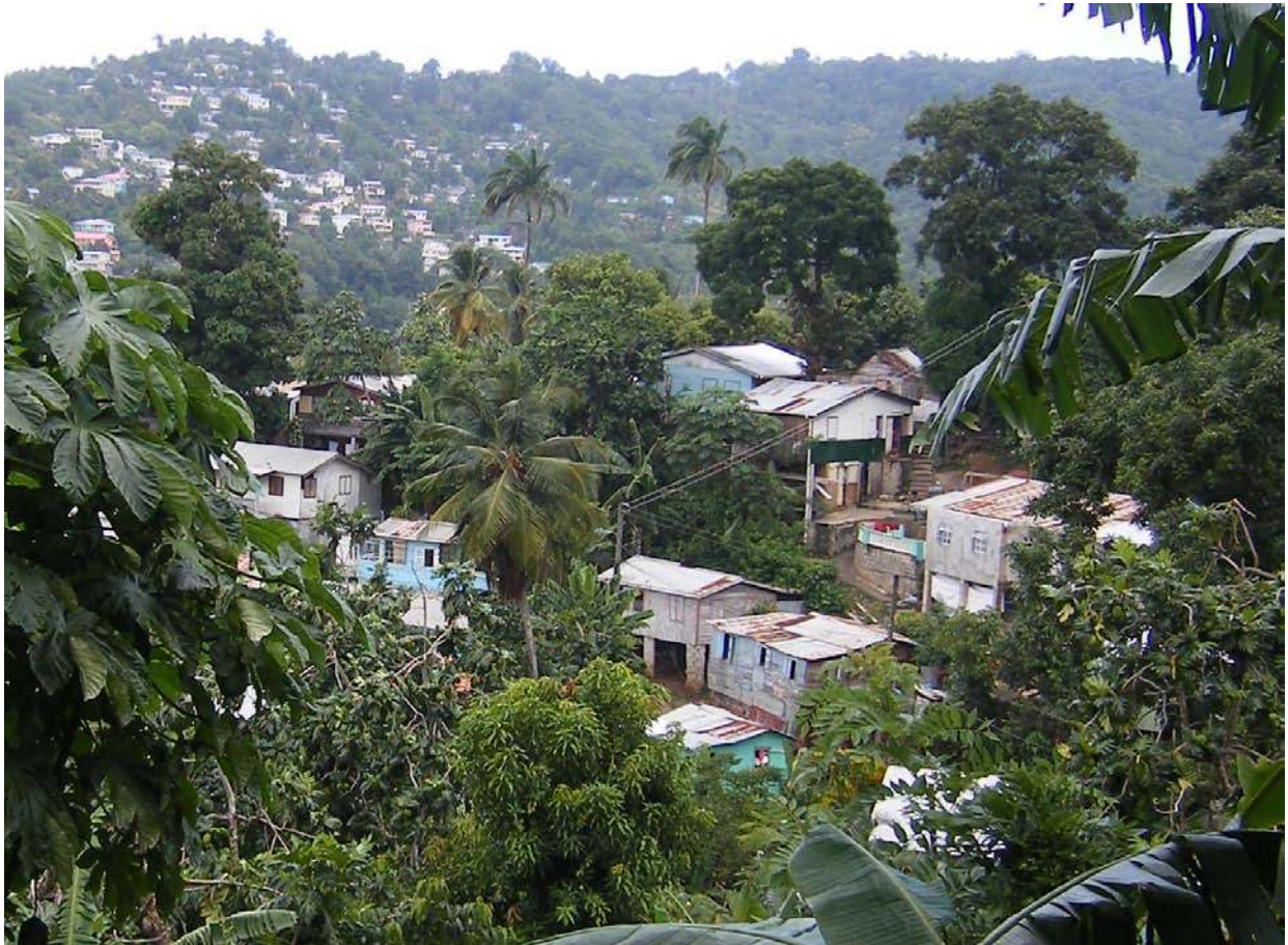
Fig. 1 Typical unplanned housing location, construction type and density in the Caribbean
