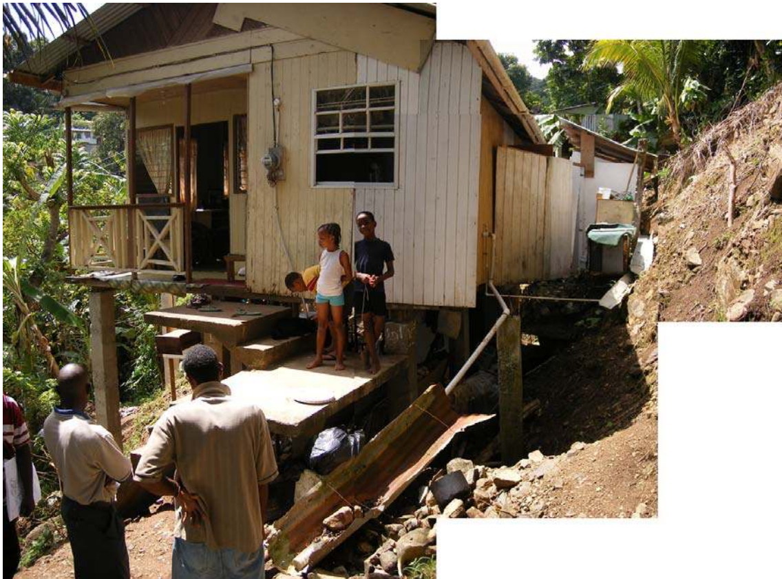
Fig. 4 Typical wooden house reconstructed (on its original site) after damage by a landslide in the cut slope above
