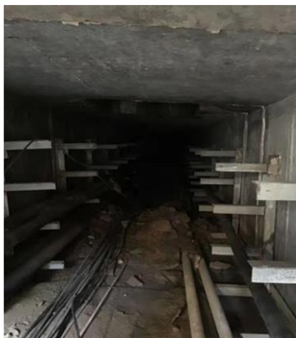
Figure 1. The real environment of the underground cable trench.
