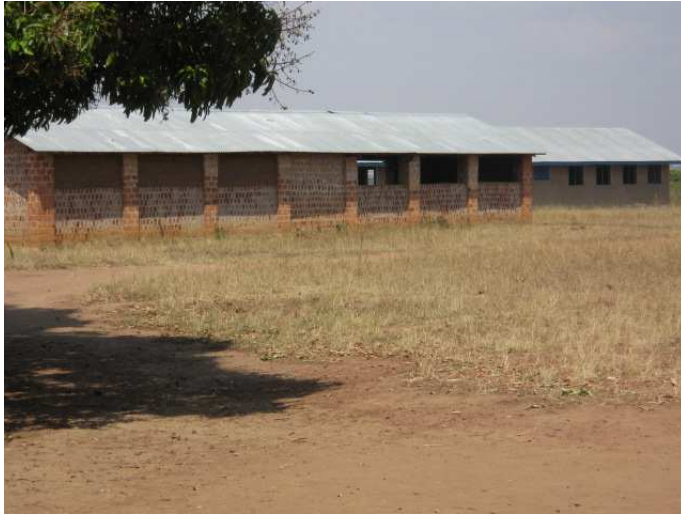
Picture 3. A UPE village school in Kamuda
