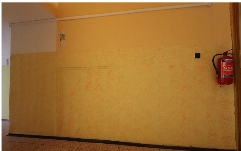
Fig. 9: Nová Horka Castle, corridor N. 211, stone portal to heater, later walled up, photo, 2021 (taken by the author).
