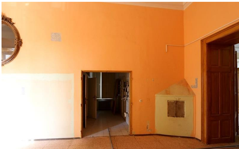
Fig. 10: Nová Horka Castle, corridor N. 231, rebuilt stone portal to the heater, photo, 2021 (taken by the author).
