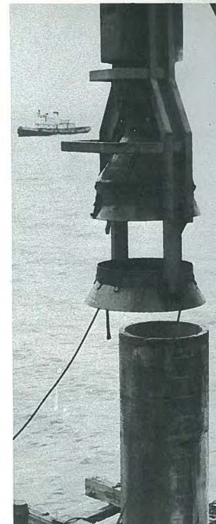
Fig. 3. Close-up of the driving of a 96-ft long 54-in. diameter cylindrical pile in 1953 for the Lake Pontchartrain Causeway. Note special driving bonnet which had to be engineered.
