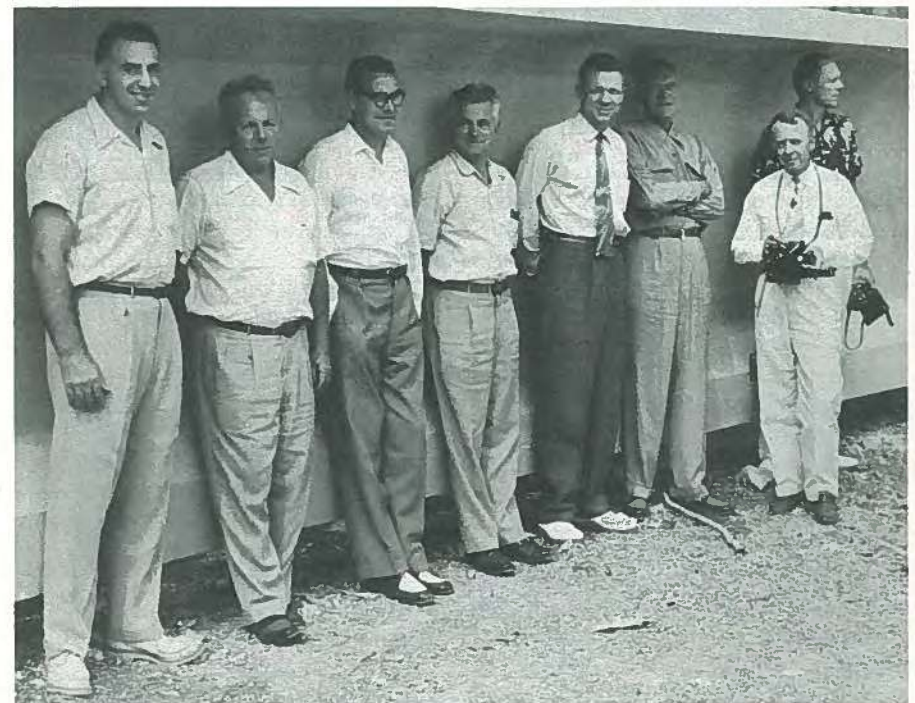
Fig. 43. The "driving forces" at Arnold Stone Co. surrounded by visiting dignitaries. From left to right: M. J. Andrews, Arnold Stone Co.; W. D. Shea, chief engineer, Arnold Stone Co.; A. Brandestini, BBR, Zurich, Switzerland; M. A. Arnold, president, Arnold Stone Co.; Millard Warren, Southern Cast Stone; Otto Formigli, Formigli Bros., Berlin, New Jersey; C. Hansen, engineer, Washington, D. C.; and Shelborne Warren, Hamilton Concrete Products.
