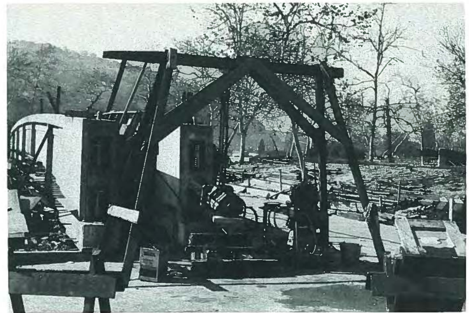
Fig. 10. Stressing the Arroyo Seco girders.
