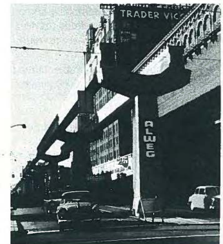
Fig. 88 View of the Seattle Monorail under construction, showing the cross section of the girders and the shape of the support columns, on a straight stretch of the beamway.
