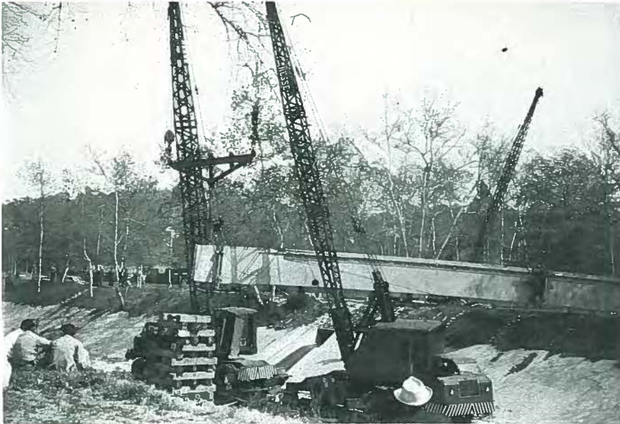
Fig. 12. The three cranes begin to lift the girders into place.
