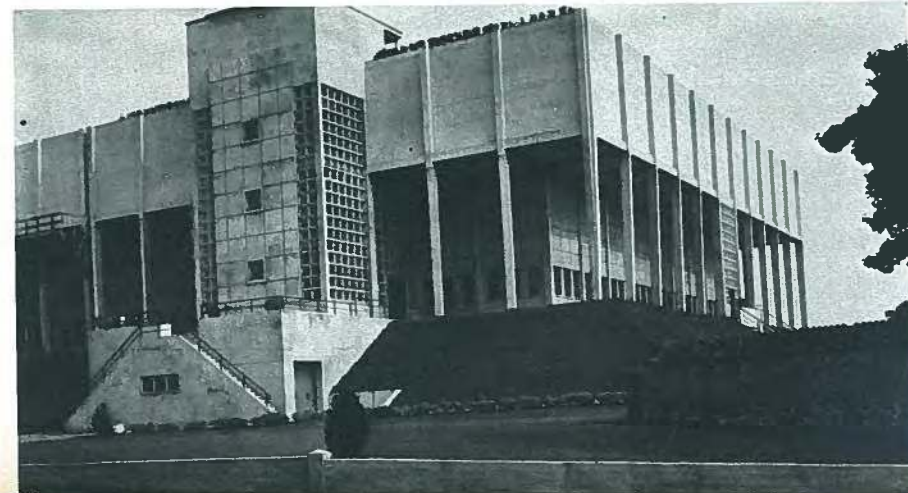
Fig. 31. Water storage reservoir and offices, Orleans, France.
