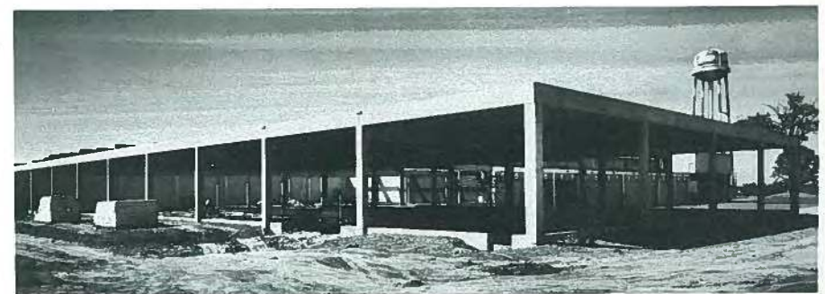
Fig. 17. One of the Cazaly/Toronto Cast Stone type of warehouses (1957).
