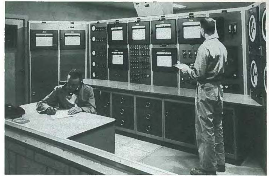
Fig. 38. Operating console in PCA's fire test center.
