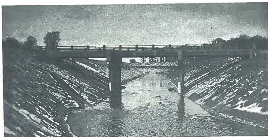
Fig. 10b. Completed three-span block-beam bridge in Tennessee.
