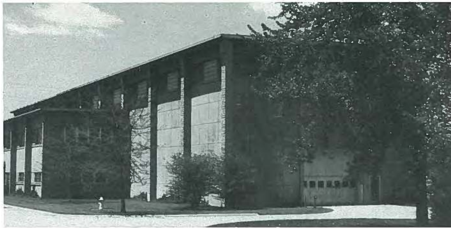
Fig. 36. PCA's fire test center.
