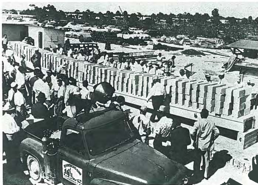
Fig. 25. Demonstration test of 100-ft (30.5 m) long prestressed channel slab at R. H. Wright & Son, Fort Lauderdale, Florida.
