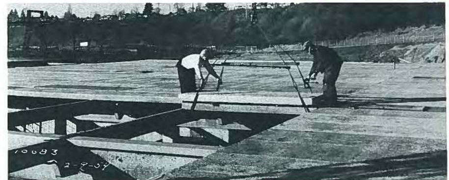
Fig. 65. Lightweight roof slabs are lowered, two at a time, into place across the structural frame. The precast slabs are 40 in. (1.02 m) wide, 10 ft (3.05 m) long and 1½ in. (38.1 mm) thick, with a 6-in. (152 mm) leg.
