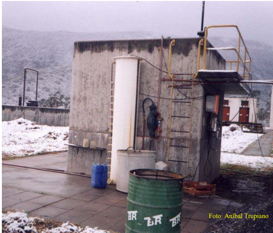
Figure 1. Pilot plant 1. Settler (not shown) and UASB reactor (white tank) on a background of “subtropical” snow.
