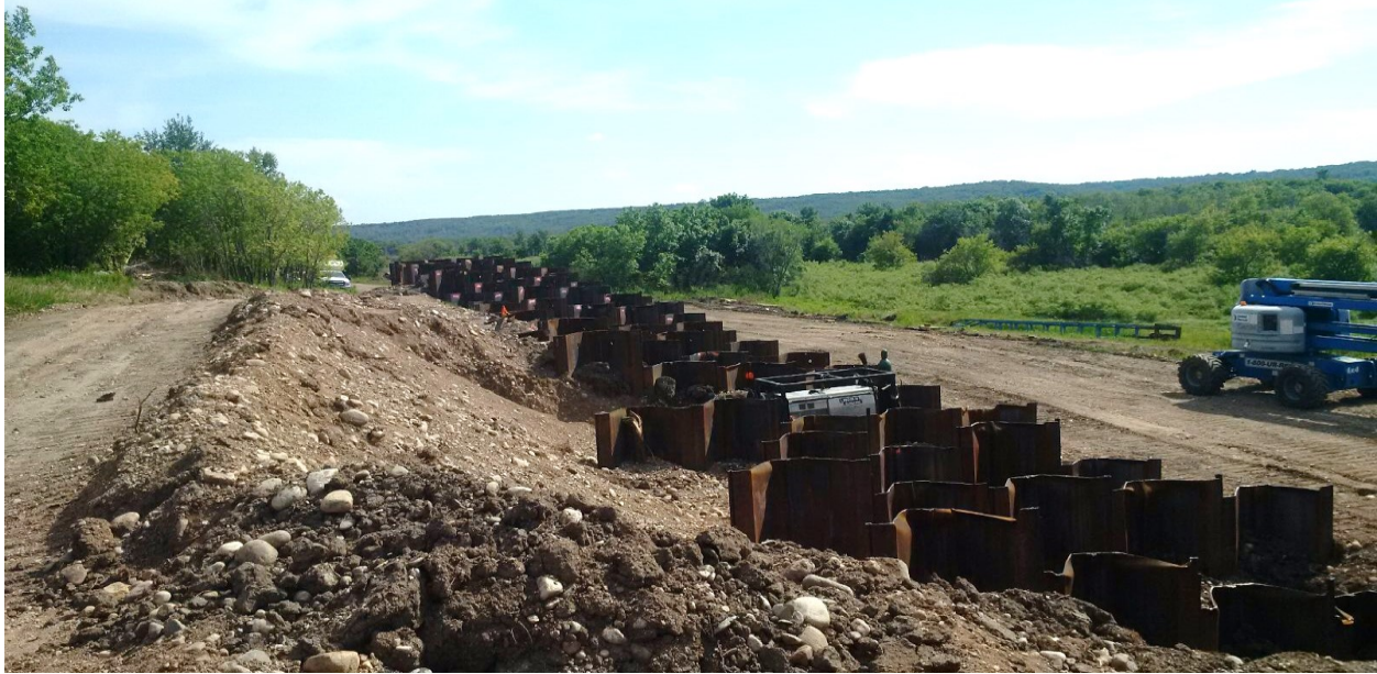
Figure 3.16: Rows of installed sheet pile walls (Source: CN).
