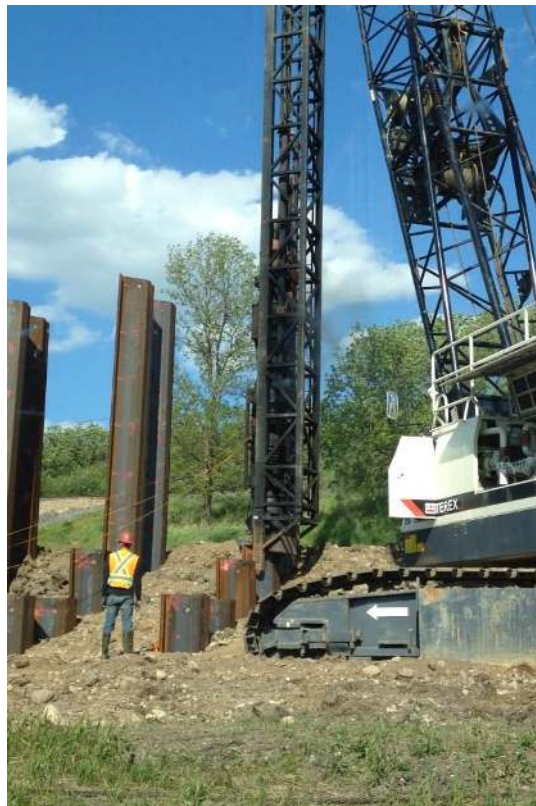
Figure 3.15: Driving sheet piles with diesel hammer (Source: CN).
