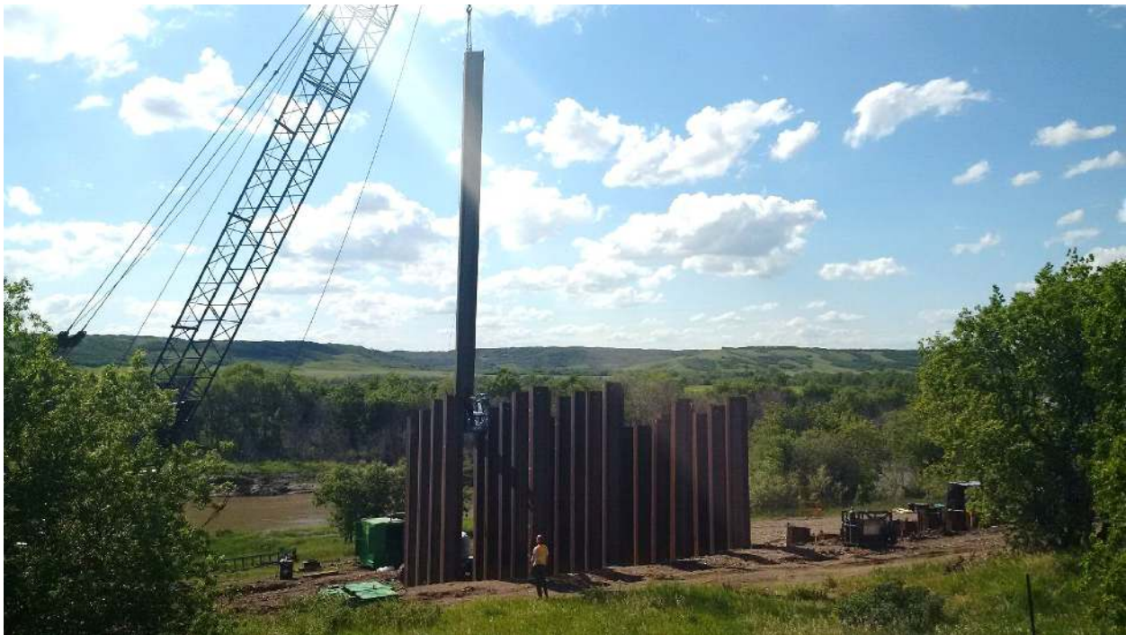
Figure 3.13: Hoisting sheet pile with crane (Source: CN).
