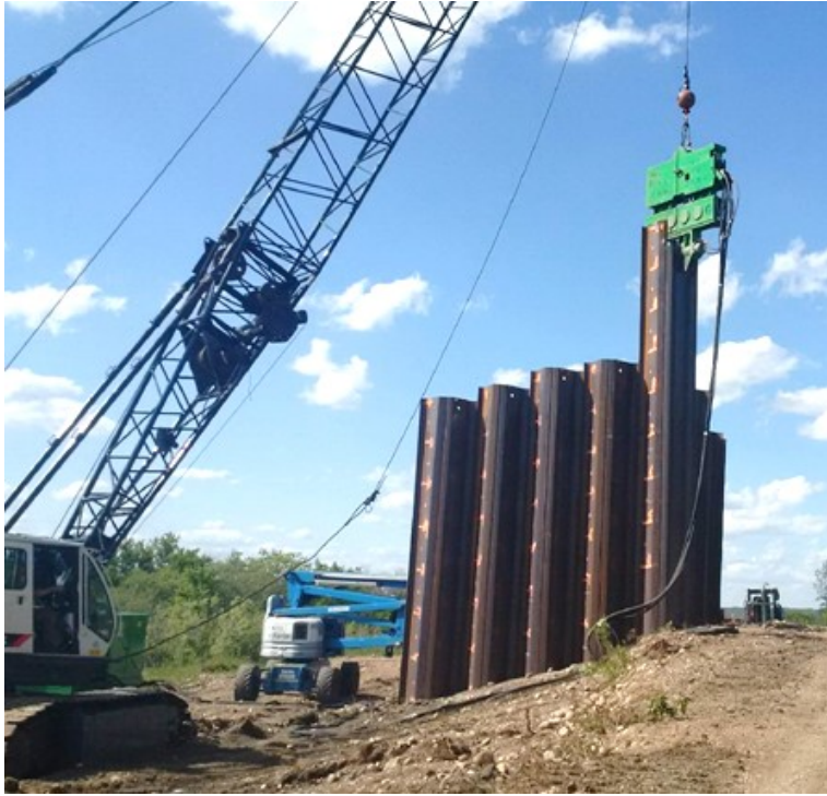
Figure 3.14: Advancing sheet piles with vibratory hammer (Source: CN).
