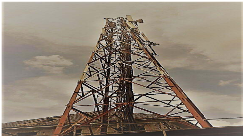
Fig. 1. Picture of MTN Mast visited at Rumuolumeni
