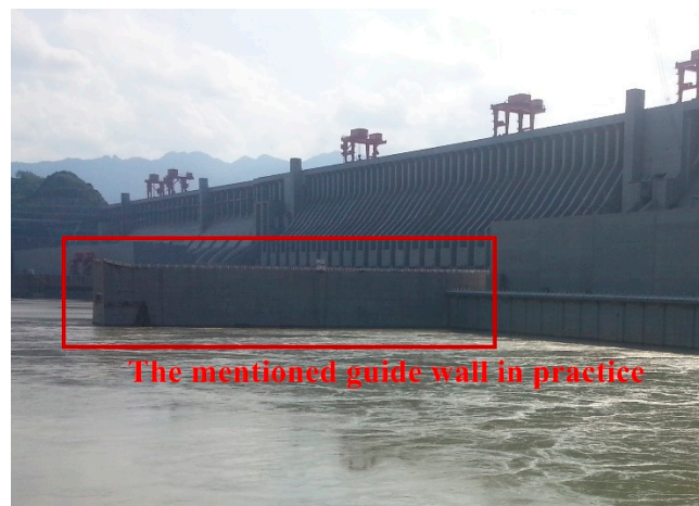
Figure 5. The left guide wall of TGHS in still water.
