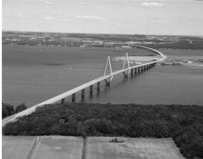
Figure 1: The Farø Bridges.
