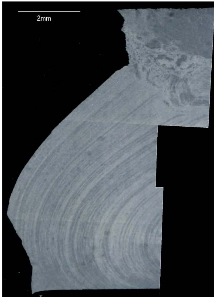
Fig. 10 Macrograph showing the fatigue crack path down through the weld region. Grain Structure of the Weld Region
