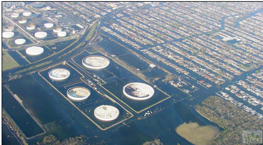
Figure 2. Flood impact in a refinery
