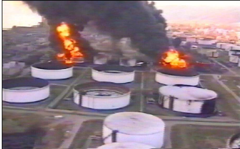
Figure 1. Fire in the refinery due to earthquakes. (Turkey, 1999)
