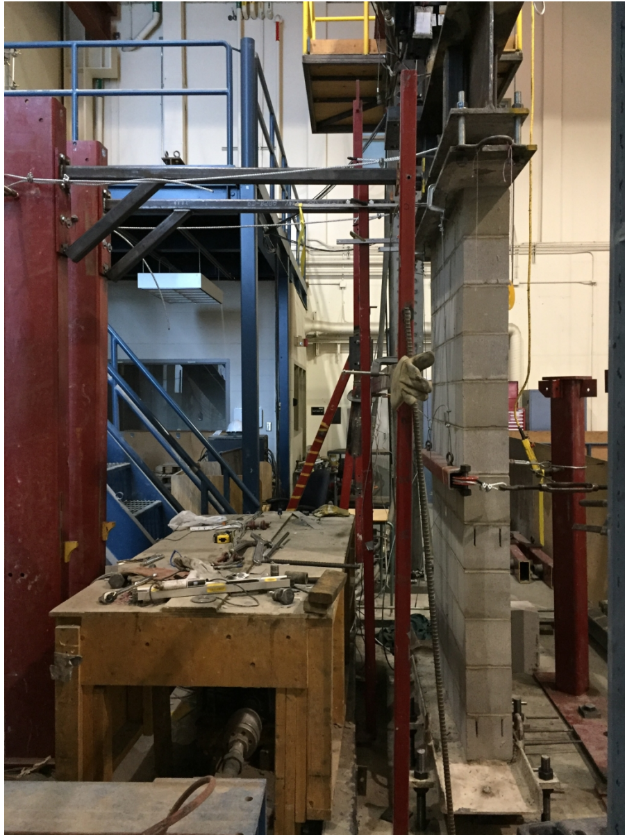
Figure 6: Vertical Section of Wall with Pinned-Fixed Supports (a) and Base Detail Showing the Wall Placed Eccentrically in the C-channel and the Steel Beneath (b)
