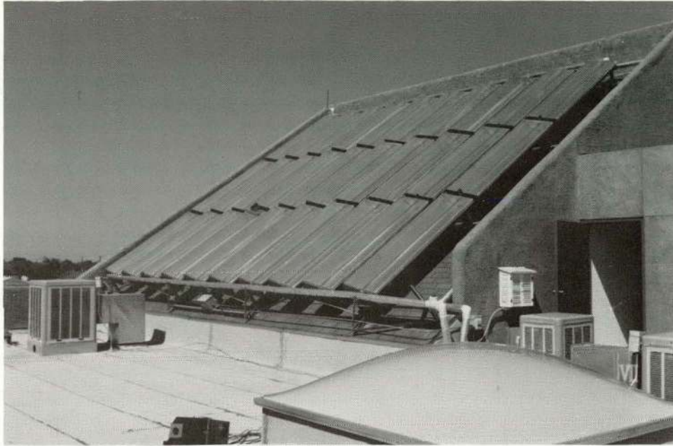
(a) View from Roof
