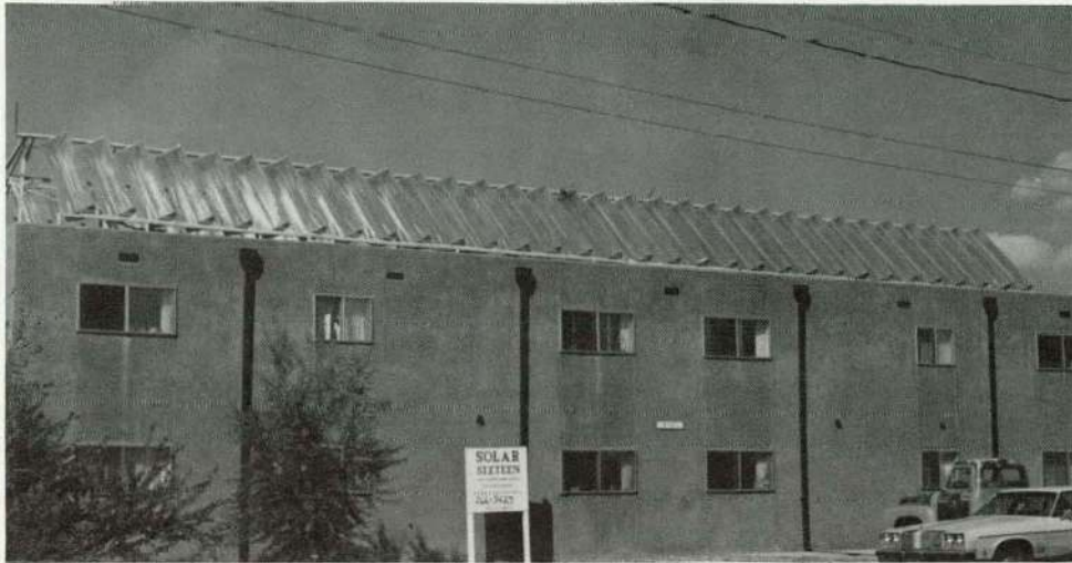
(a) View from Street
