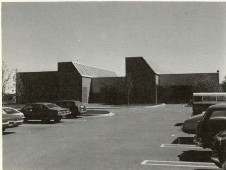
(a) Overall View
