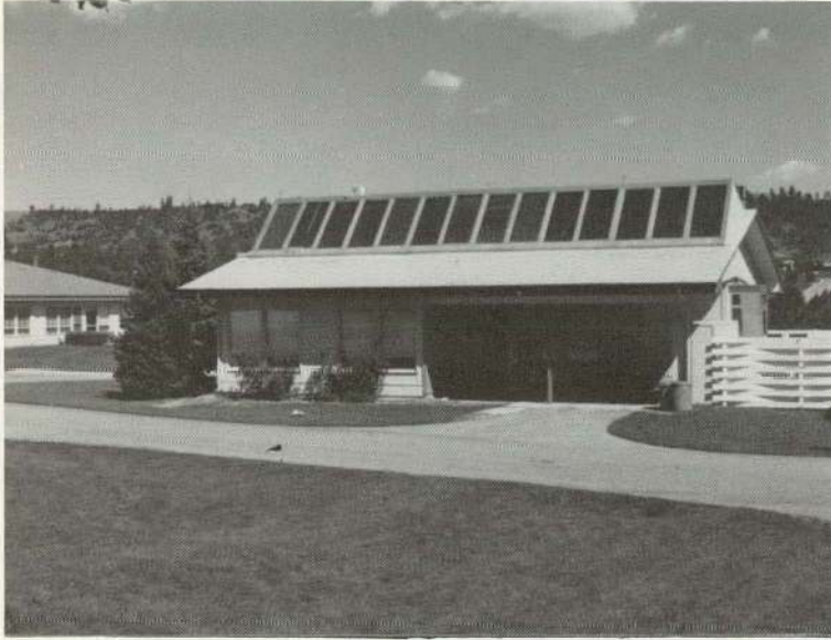
(a) Roof Array
