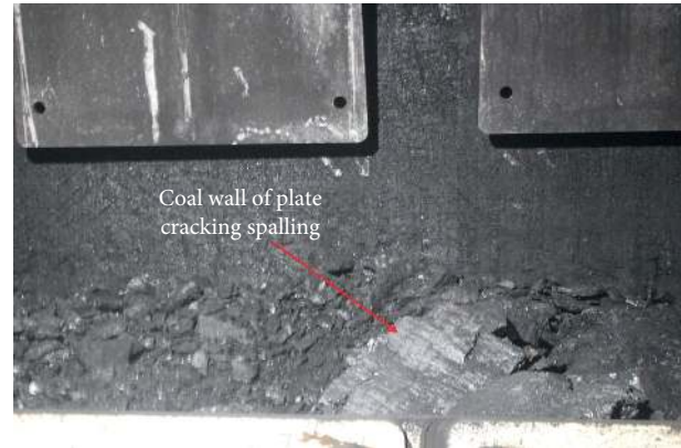
FIGURE 3: Plate cracking phenomenon in Jinjitan coal mine, China.
