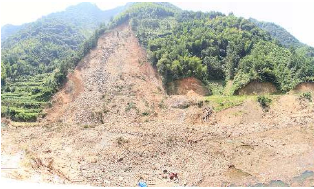
Figure 4. The scene of the Tangjiaxi landslide, taken on 23 July 2014, when the water level was 167 m a.s.l. The river was full of wood and debris, which were the destroyed building materials.
