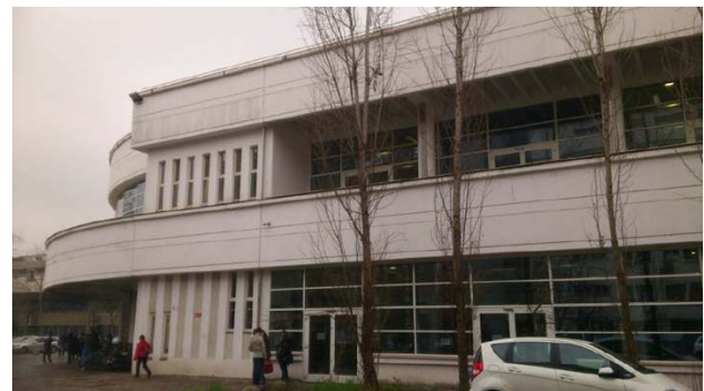
Fig. 2 View of north façade of the building
