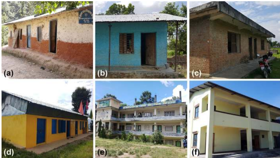
Fig. 1 School building typologies: a Stone-mud masonry [URM-SM], b brick-mud masonry [URM-BM], c brick-cement masonry [URM-BC], d metallic with masonry infill [S], e non-engineered RC [RC-N], f engineered RC [RC-E]. Source SAFER-App database, University of Bristol (Sextos and Mason 2018)
