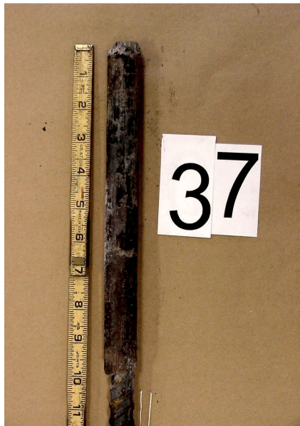
Figure 7. View of a short column grout anchor recovered from the roof.
