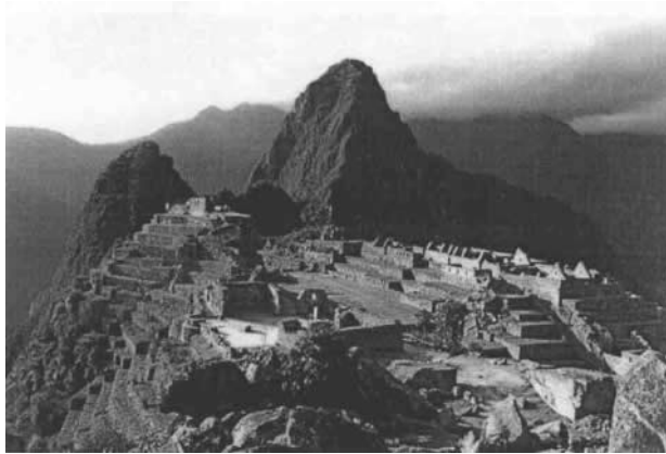
Figure 1. Machu Picchu Was in Good Condition after Four Centuries of Rain Forest Growth When Discovered by Yale Explorer Hiram Bingham in 1911. Its Longevity and Resistance to Landslides and Settlement Are Result of Extensive Drainage Systems Built by Inca in 15th and 16th Centuries.
