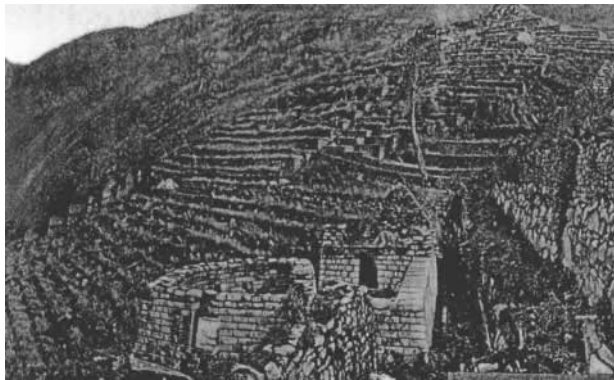
Figure 2. Hiram Bingham's 1912 Photo of Machu Picchu Agricultural Terraces Showing Hundreds of Undamaged Stone Walls That Resisted Landslides and Earthquakes. Surface and Subsurface Drainage Works Were Built to Handle 1,940 mm of Average Annual Rainfall. Temple of the Sun Is Shown in Foreground with Its "Most Beautiful Wall" Intact on Right (Bingham 1930).
