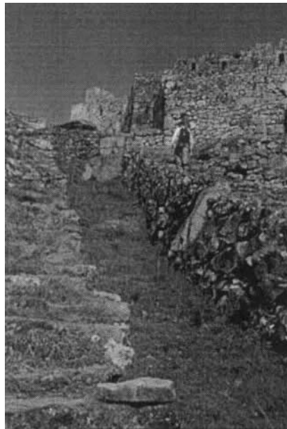
Figure 8. Main Drain of Machu Picchu, Sometimes called the Dry Moat, this Drain Overlaid Local Geologic Fault. Main Drain Discharges into Rainforest Below. Effective Engineering Layout of Drainage Infrastructure Was Main Element in Longevity of Machu Picchu.
