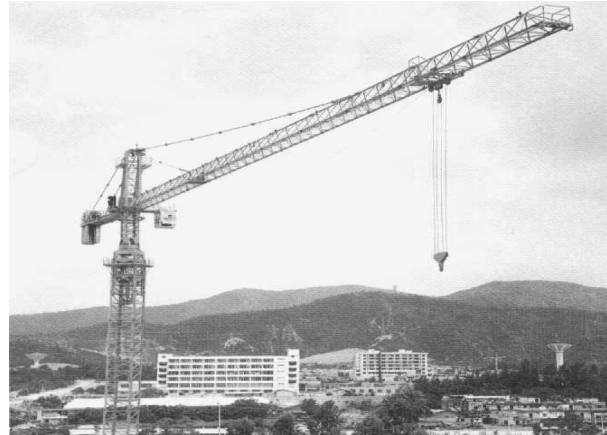
(b) Tower crane.
