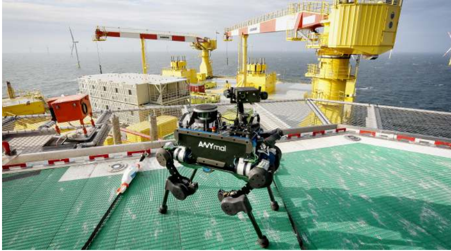
Fig. 1: The quadrupedal robot ANYmal was deployed for autonomous inspection and surveillance on a wind energy HVDC converter platform in the North Sea.
