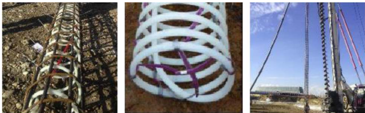
Fig. 21 Spiral borehole heat exchanger [16]
