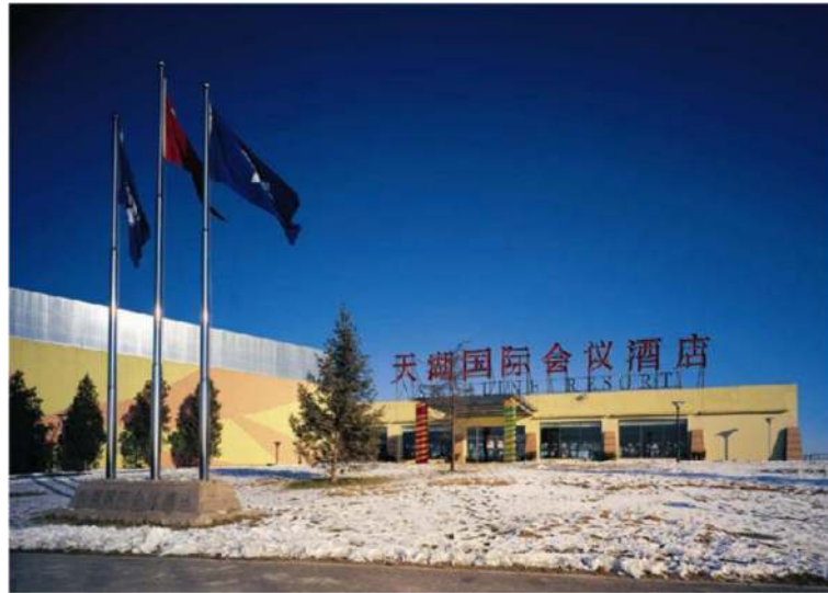
Fig. 15 Beijing Tianhu International Conference Hotel
