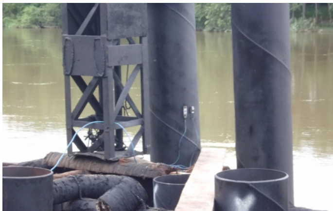
Figure 1. Example of installed accelerometer (right) and strain transducer (left) on the pile.
