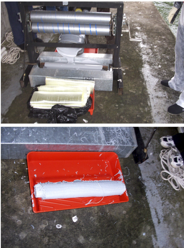
Fig. 8. On-site saturation of fiberglass fabric.
