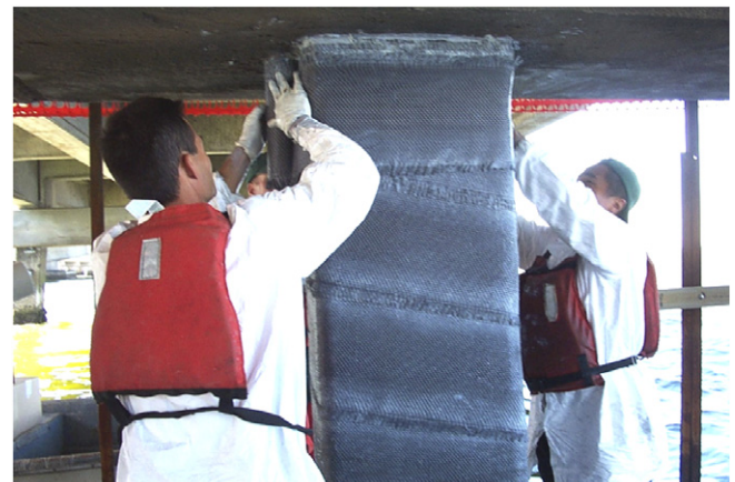
Fig. 7. Applying second transverse CFRP layer.
