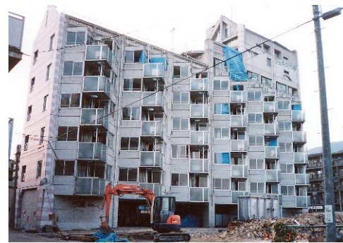
(a) View of RC frame-structure building
