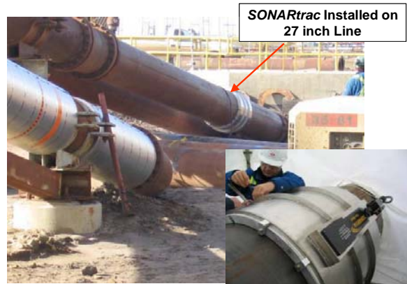
Figure 10: Installation of Sonar-based flow meters on 27inch commercial hydrotransport line
