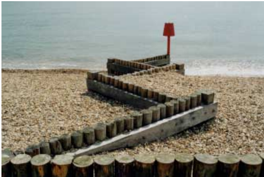
Figure 30. Low cost groyne at Calshot, UK
