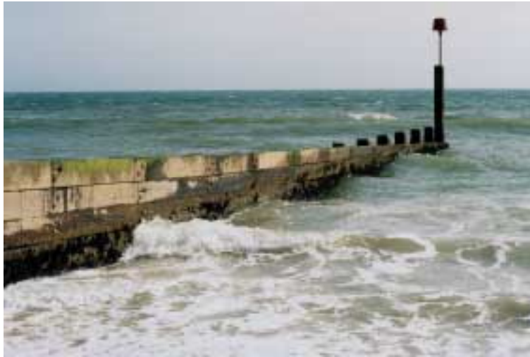
Figure 3. Conventional impermeable timber groyne (Bournemouth, UK)
