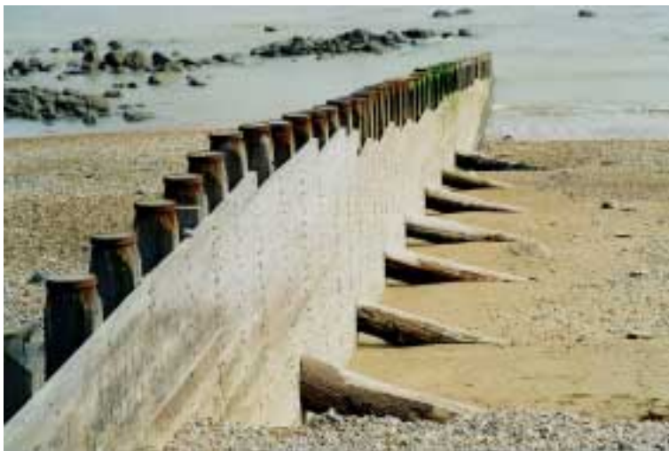
Figure 1. Timber groyne (Eastbourne)
