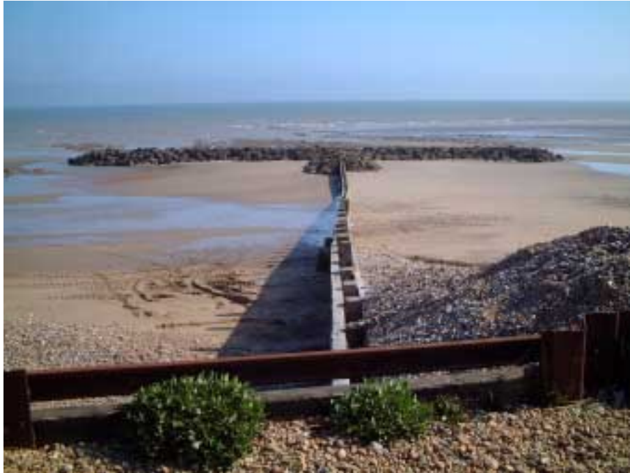
Figure 60. Combined use of rock and timber
