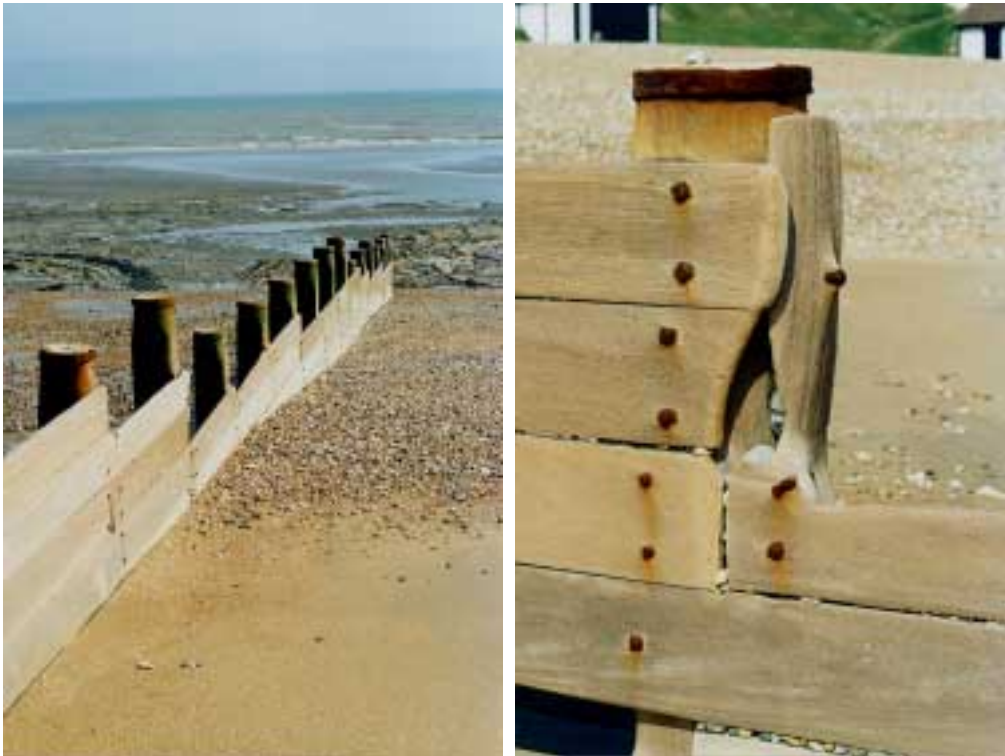
Figure 24. Groyne at Bexhill with underlying bedrock showing at low tide
