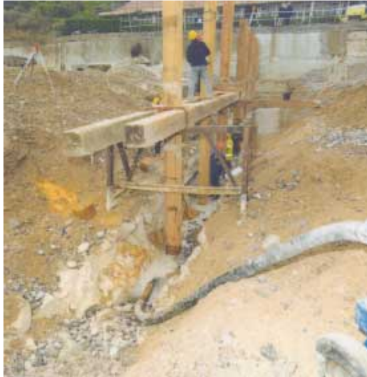
Figure 26. Planting posts in trench (courtesy to Posford Haskoning)
