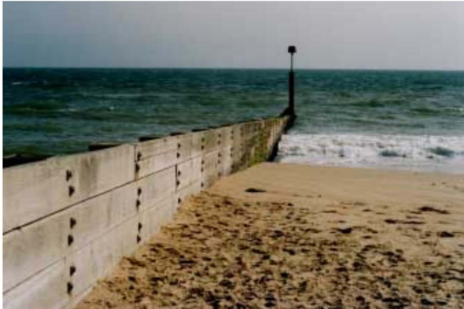
Figure 27. High quality groyne at Bournemouth
