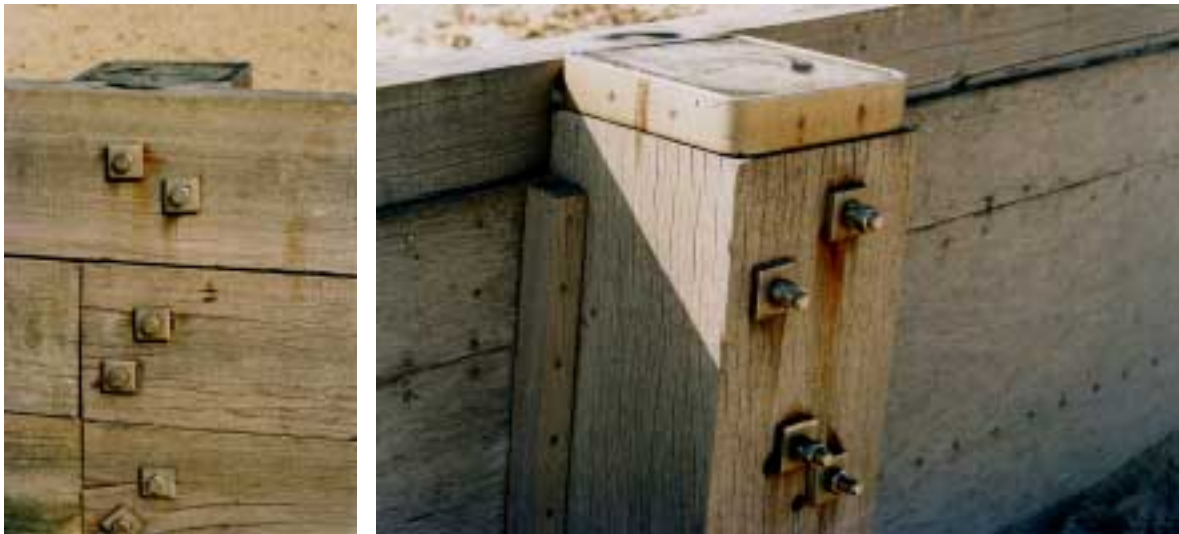
Figure 28. Stainless steel fixings and pile rings
