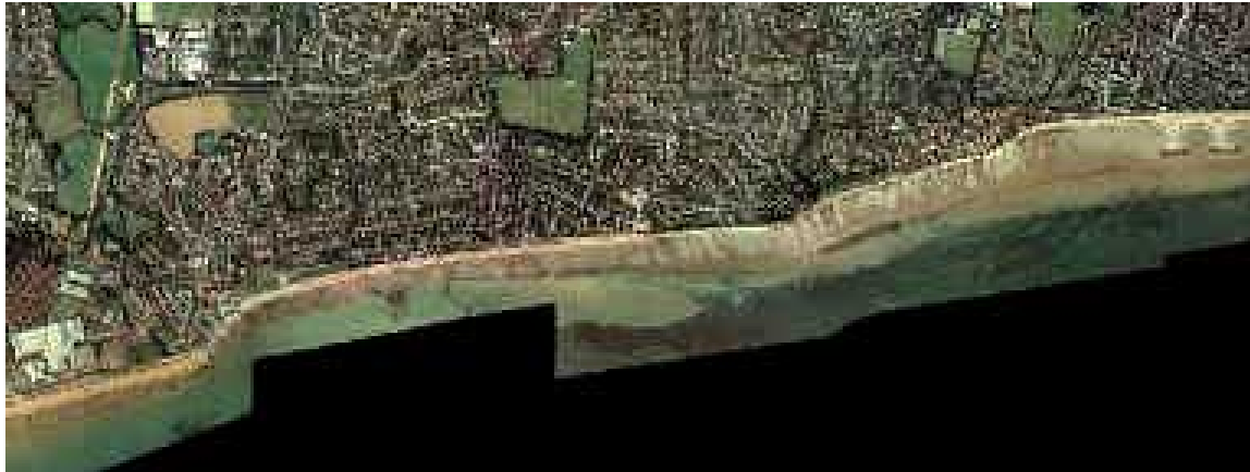
Figure 73. Aerial photograph of Felpham scheme (courtesy to Multimap)
