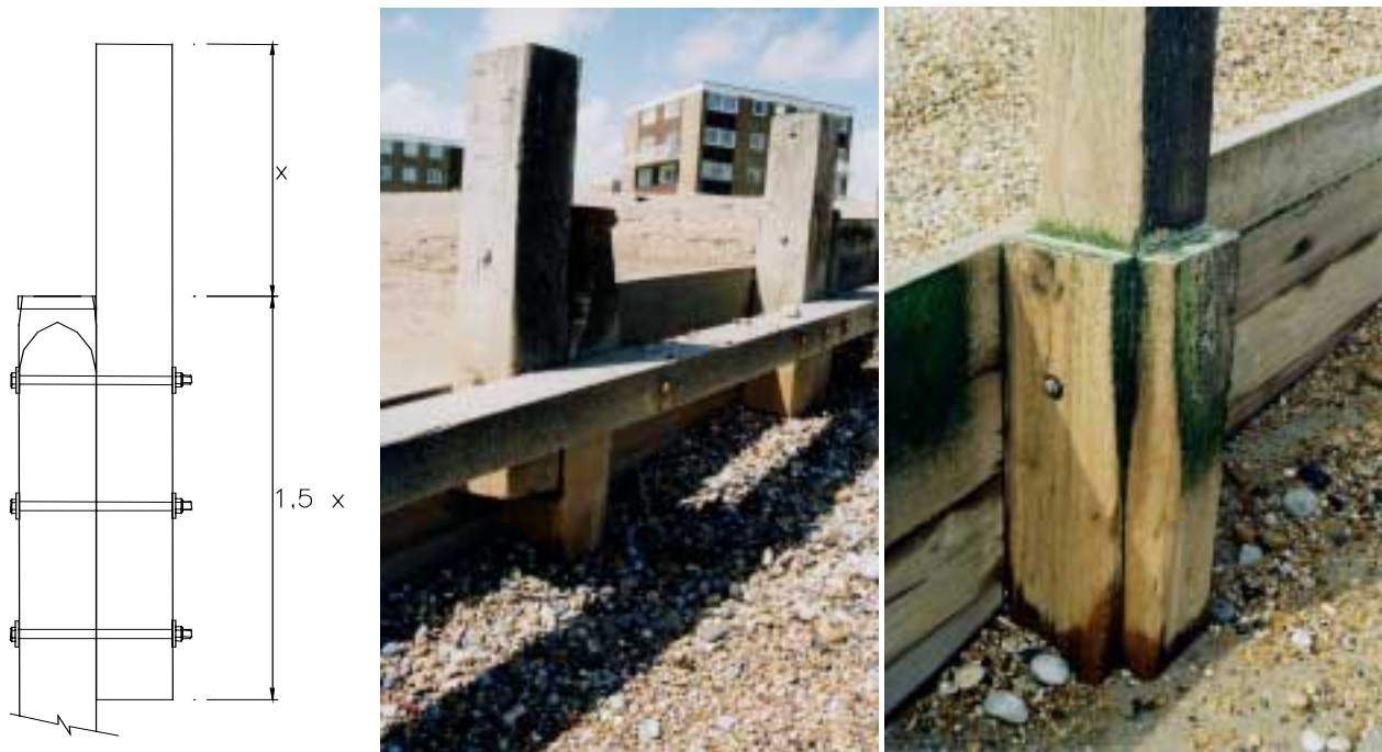
Figure 58. Pile extension Figure 59. Rubbing pieces
