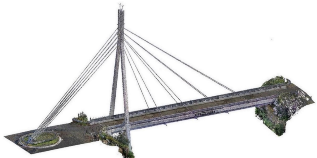
Figure 6. Generated point cloud of Werrington bridge.
