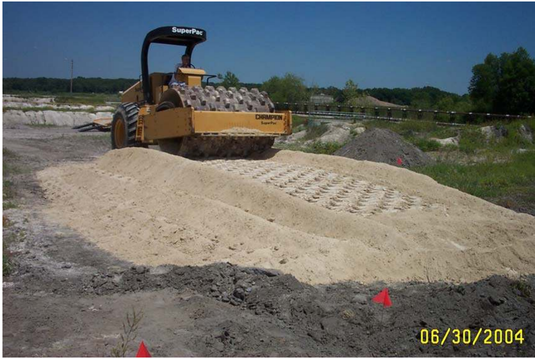
Figure 60: Compacting the test embankment
