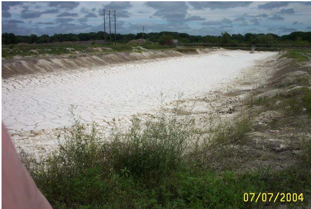
Figure 3: Dewatering Lagoon after 10 Months Settling
