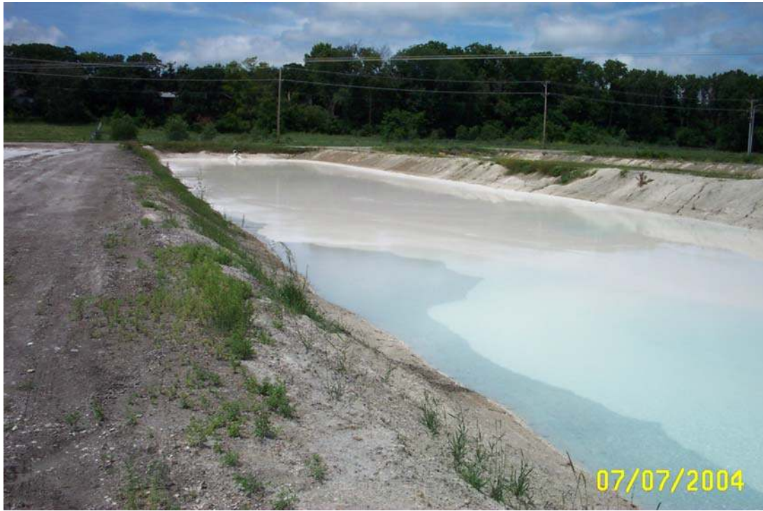
Figure 1: Dewatering Lagoon While Filling
