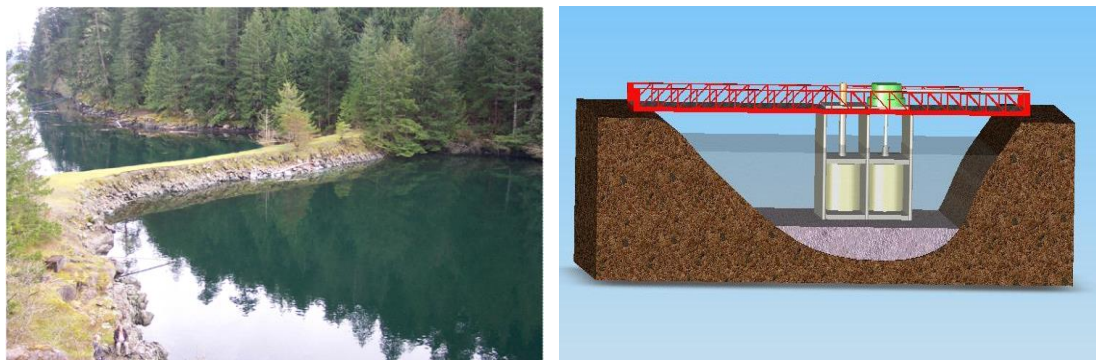
Figure 6. Photo (left) showing existing rock dam and depicted graph (right) showing replacement of the dam with two underwater turbines.
