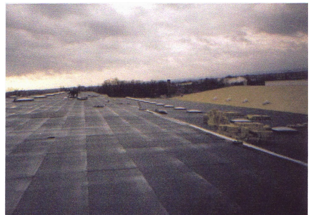
Fig. 1. The roof on the developed object Kunice
